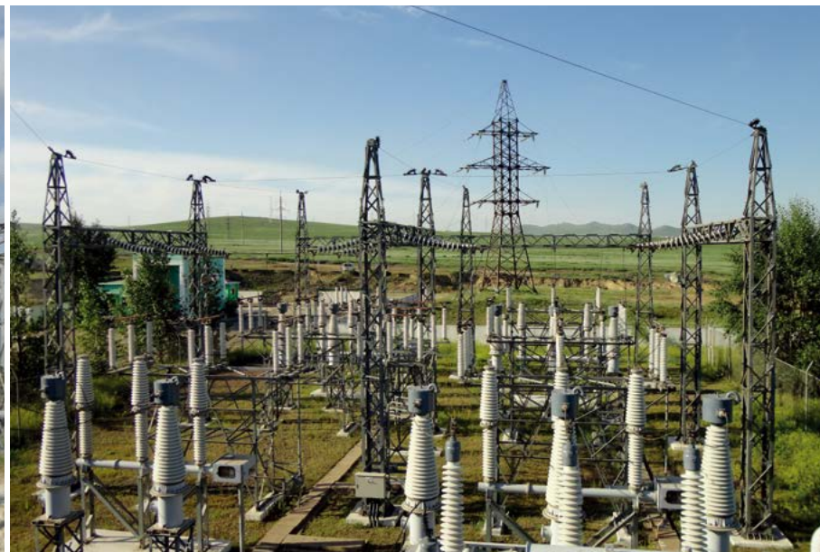
132 kV DMP Substation for Mongolia
