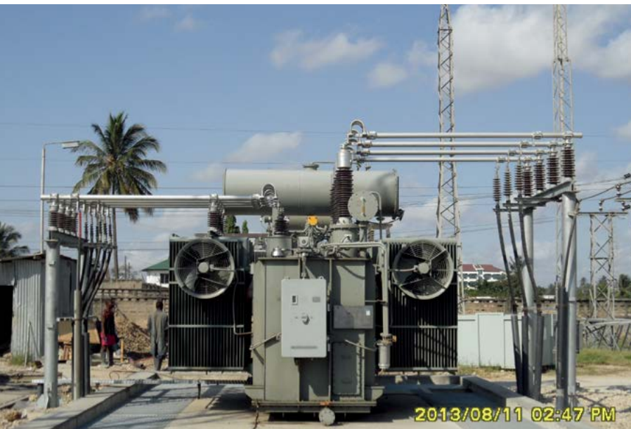
132/33/11 kV Transformers for Ubungu Substation in Tanzania
