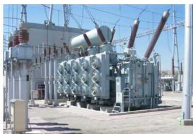
220kV Transformer
