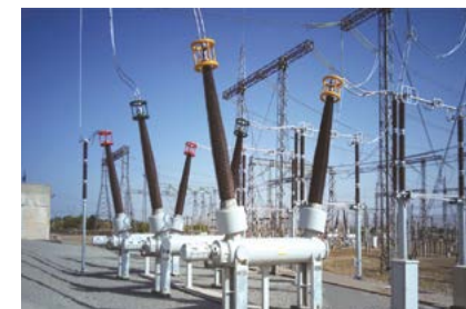
550kV DT Circuit Breaker for Tajikistan
