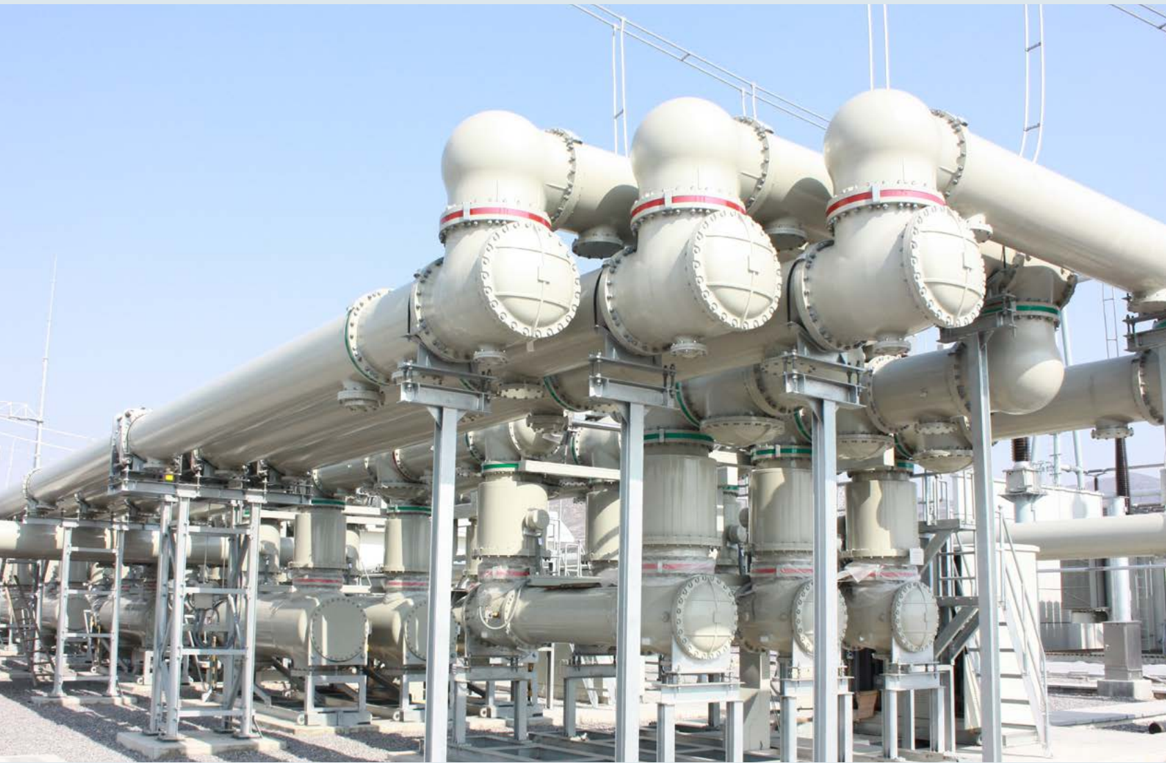
550 kV GIS for Xinduqiao , a smart substation with the highest altitude of 3,600m in China
