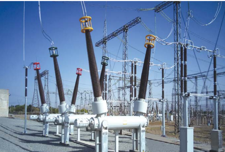
550kV DT Circuit Breaker for Tajikistan
