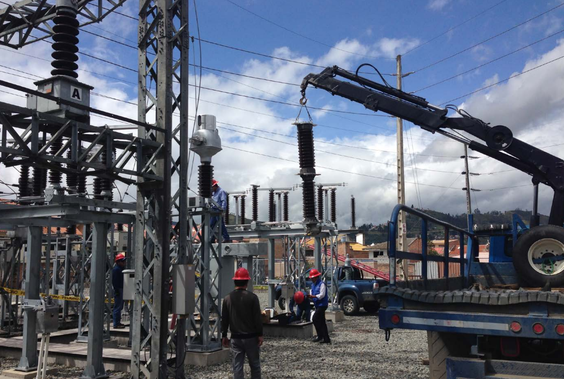
Taikai EPC turnkey projects offers you great efficiency
