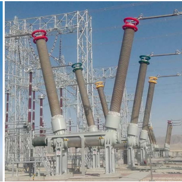
800kV Circuit Breaker
