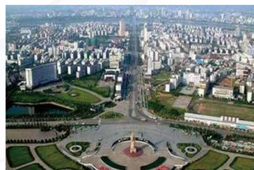
The urban intelligent lighting at Chaling county, Hunan province
